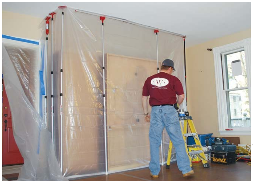
ZipWall and Woodway Renovations
