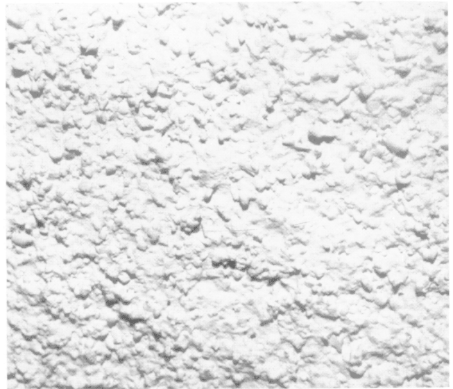
Friable, cementitious sprayed-on or troweled material (acoustical plaster)
